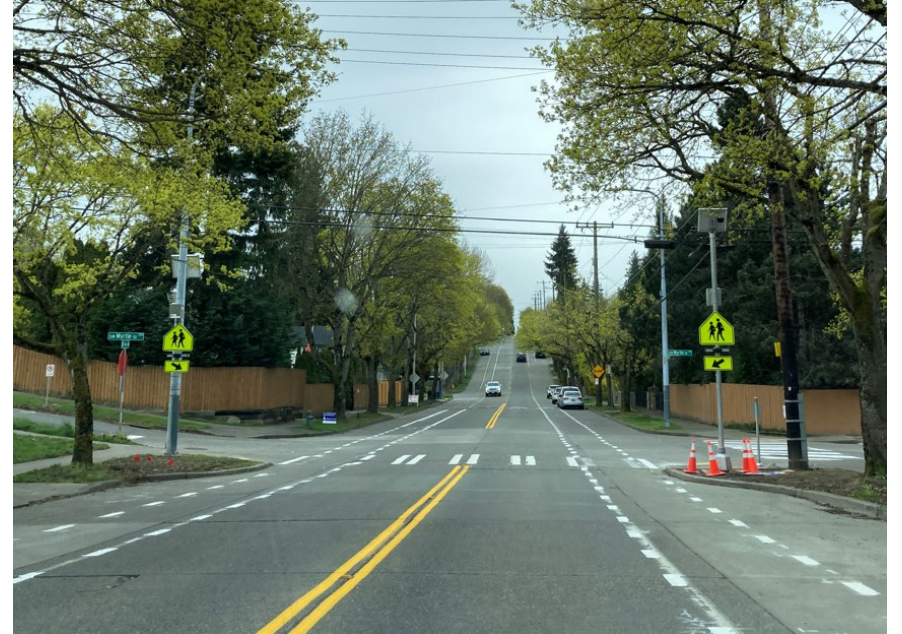
16 th Ave SW and SW Myrtle St Rectangular Rapid Flashing Beacon (RRFB)
