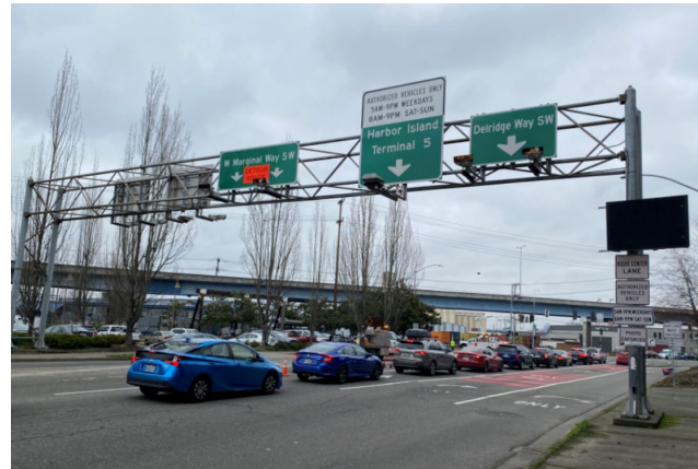
Overhead signage replacement
