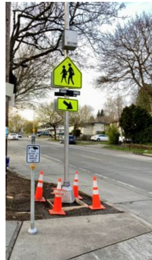
RRFB at 16 th Ave SW and SW Myrtle St
